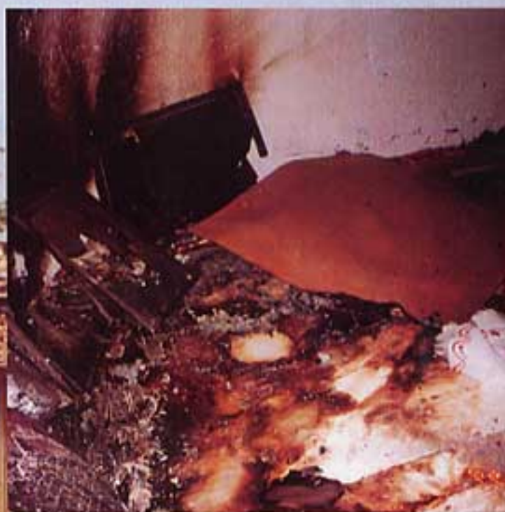
Damaged church of St. Elijah Повреждения храма.
