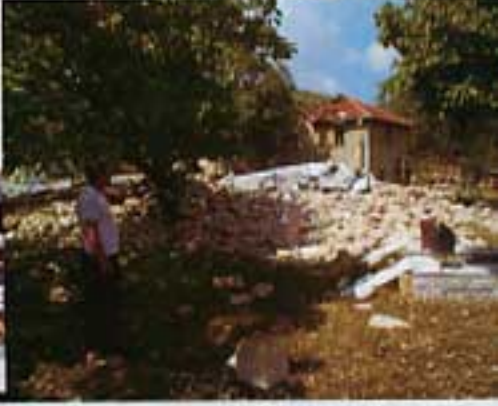
The church after destruction Храм после взрыва.
