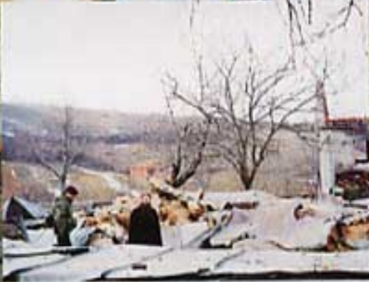
The church after destruction Храм после взрыва.
